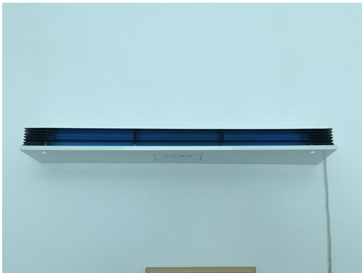
Figure 2. Upper-level ultraviolet germicidal lamp (UVGI)
